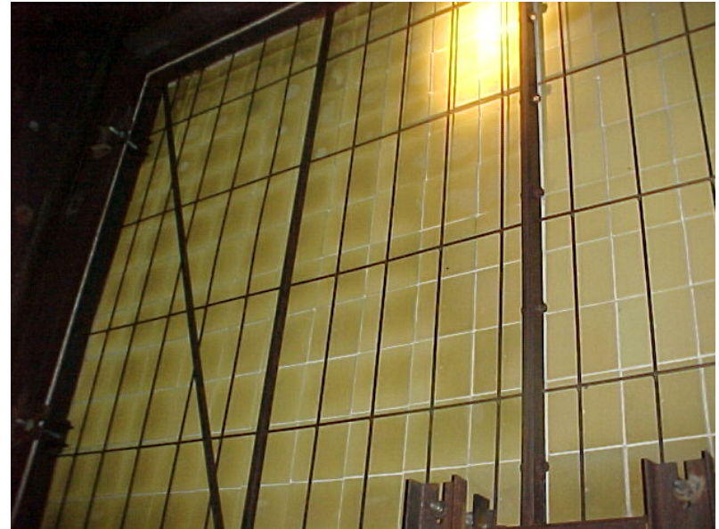
Commercial Scale SCR installation
